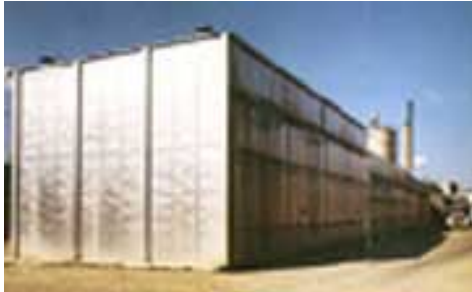
Lumber Mill Energy Plant
